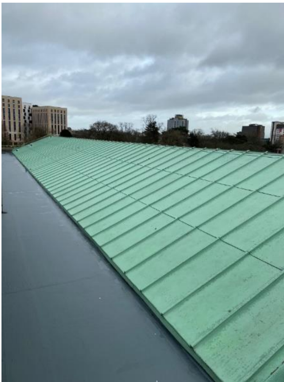
New Copper Roof over the Main Hall, Jan 2023
